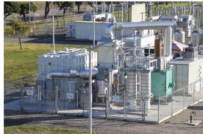
2.4-MW biogas fuel cell plant in San Diego
