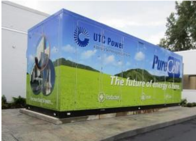
400-kW hydrogen fuel cell plant in Connecticut
